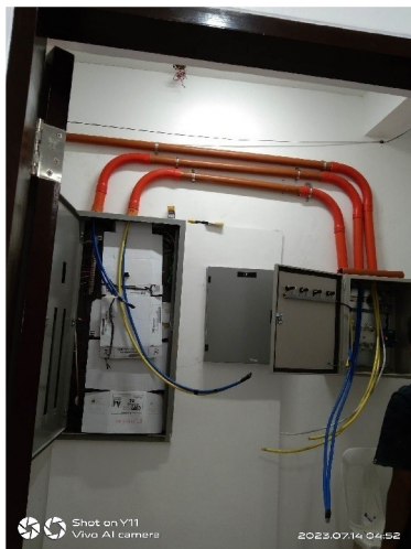
A. Cable Pulling and Terminations of sizes ranging from 14sq.mm up to 200 sq.mm, Panelboard & Devices Assembly and Installation
