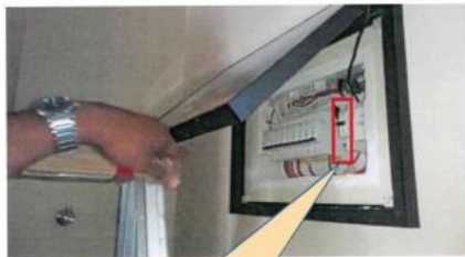
Only the refrigerator CB is on ON position, energized and now fed from 63A MCCB
