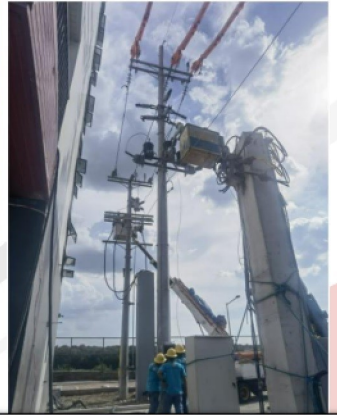
SUPPLY, INSTALLATION, COMMISSIONING AND ENERGIZATION OF 3-MVA PAD-MOUNT TRANSFORMER (OHPM) 3-PARTS 12-STOREY MIXED USE PROJECT, KAWIT CAVITE
