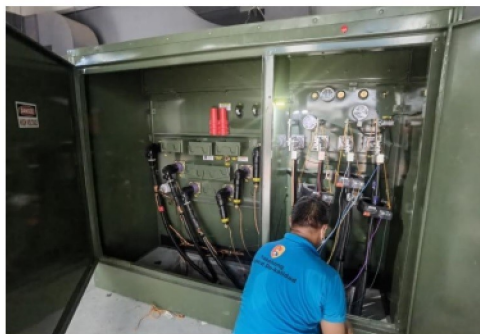
\Delta - Y_6 or Y - Y_6 PAD MOUNT TRANSFORMERS UP TO 2MVA
